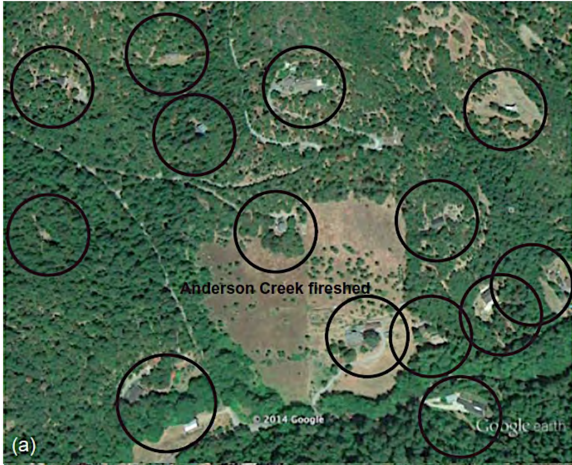
Fig. 3. Google Earth image of the Anderson Creek watershed (southwest Oregon) and community fireshed showing a housing development. Circled areas depict where proper fire risk reduction has the greatest chance of saving homes in a fire 11 .
