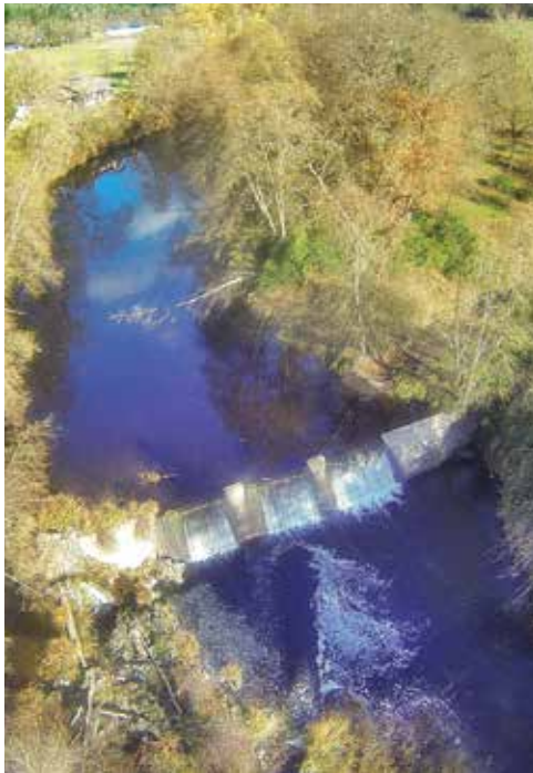
Wimer Dam before removal, Evans Creek
