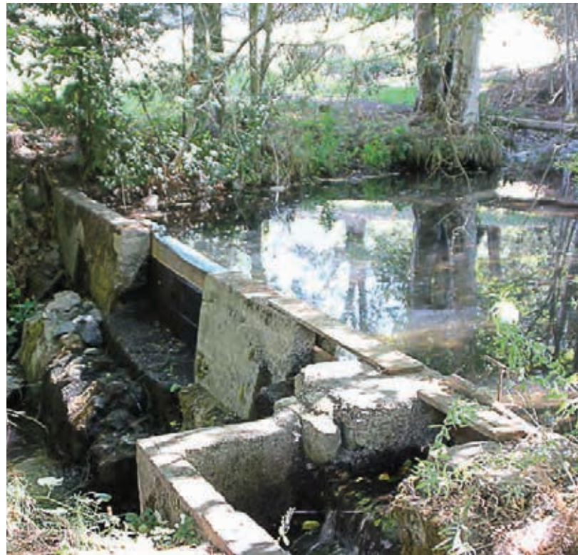
Wagner Creek water diversion
